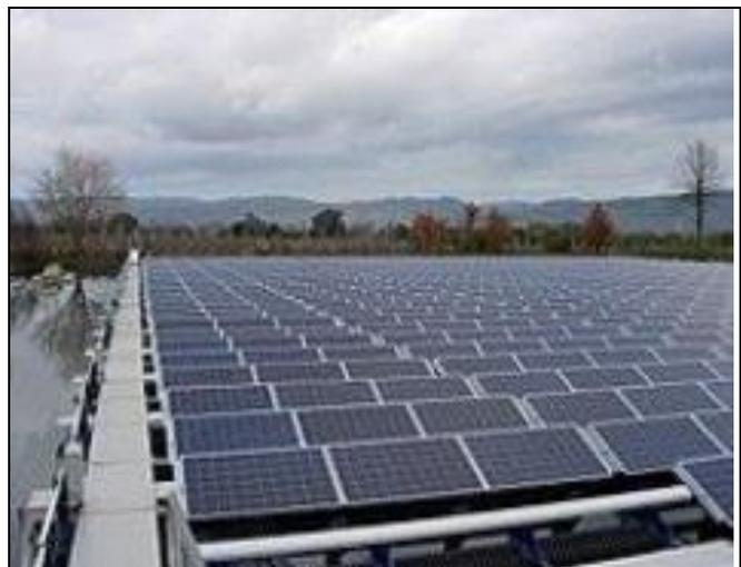
Fig 5 Floating Photovoltaic on an Irrigation Pond
