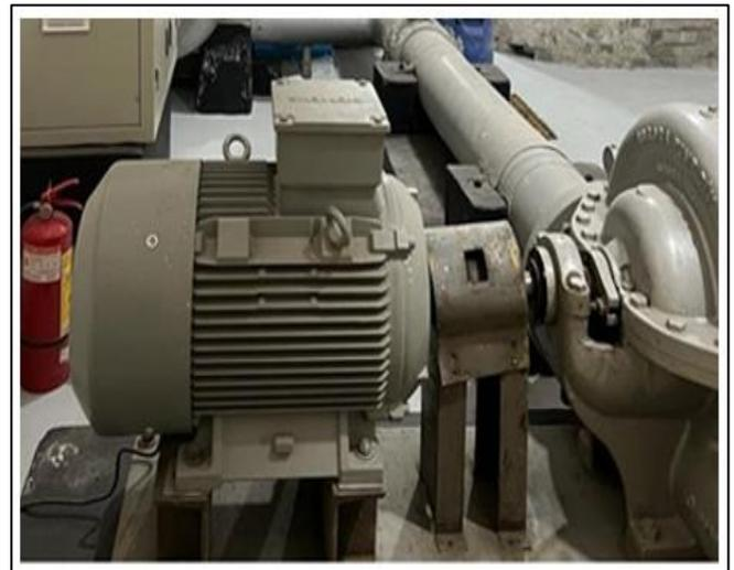
Fig 11 Newly Replaced Primary and Secondary Pump Motor of BTRR
