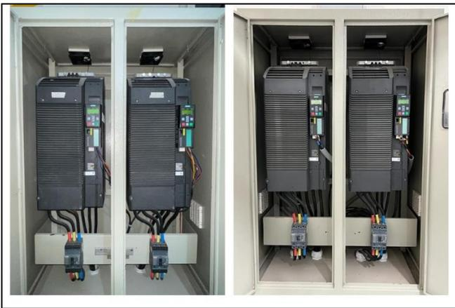
Fig 10 VFDs for Primary and Secondary Pumps of BTRR
