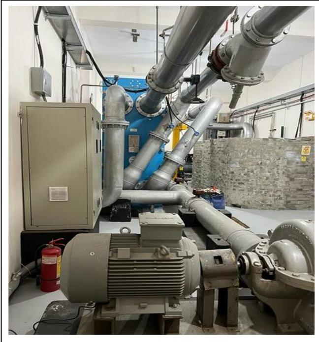
Fig 3 Piping Network of BTRR Colling System.
