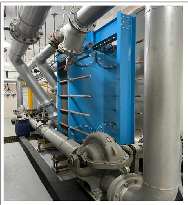
Fig 4 Heat Exchanger of BTRR Colling System
